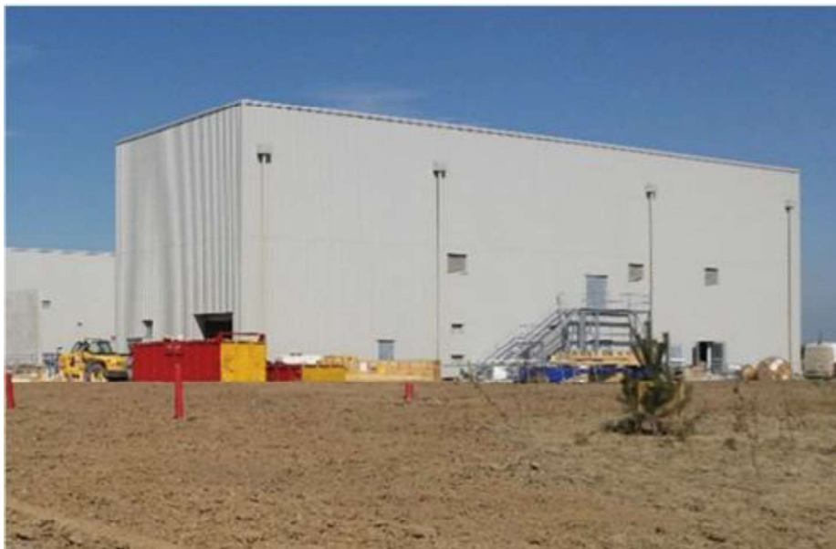
Figure 5.6: Typical 220kV GIS Substation Building
